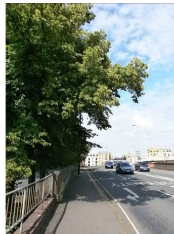
Photo 2.6: Looking north along Central Bridge
